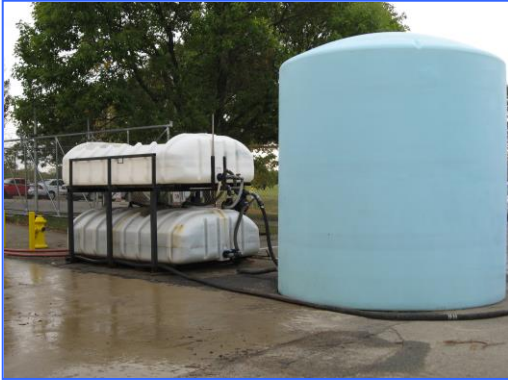
Figure 44: Brine used for road deicing. Like road salt, salt brine is a pollutant to streams and should be stored indoors or in secondary containment. Loading truck tanks with brine should be performed indoors, on grass, or away from storm drains. 44
