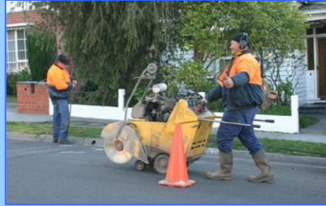
Figure 25: A concrete saw. Concrete saws are frequently used in road maintenance activities and can be a large source of stormwater pollution if precautions are not taken. 25
