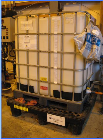
Figure 31: (left) A containment pallet under a liquid storage unit. Containment pallets are useful in preventing slow leaks from spilling onto the floor or ground. They are not useful for large breaches in primary containers. 31
