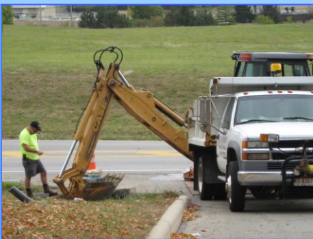
Figure 27: (left) An example of dredging near a road. A Pollution Prevention/Good Housekeeping technique in this case would be placing a mat over nearby storm drains or temporarily berming the work area or storm drain (putting a barrier around
