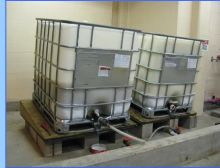
Figure 31: (left) A containment pallet under a liquid storage unit. Containment pallets are useful in preventing slow leaks from spilling onto the floor or ground. They are not useful for large breaches in primary containers. 31
