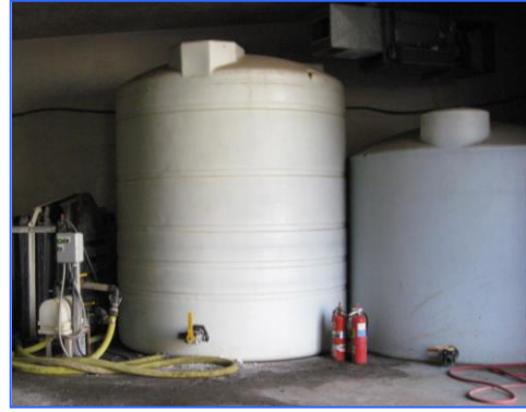
Figure 44: Brine used for road deicing. Like road salt, salt brine is a pollutant to streams and should be stored indoors or in secondary containment. Loading truck tanks with brine should be performed indoors, on grass, or away from storm drains. 44
