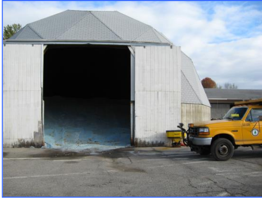
Figure 42: Road salt storage. Road salt or deicers should be stored in covered shelters with a door. Although road salt is spread liberally on roads for safety, it is important that we limit the amount of stored road salt that enters streams. Protecting stored road salt from the elements (wind or precipitation) saves money since very little is wasted and keeps unnecessary salt out of our streams. 42
