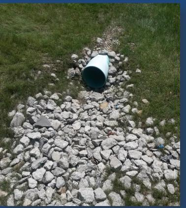
Still need erosion/scour protection at basin inlet.
