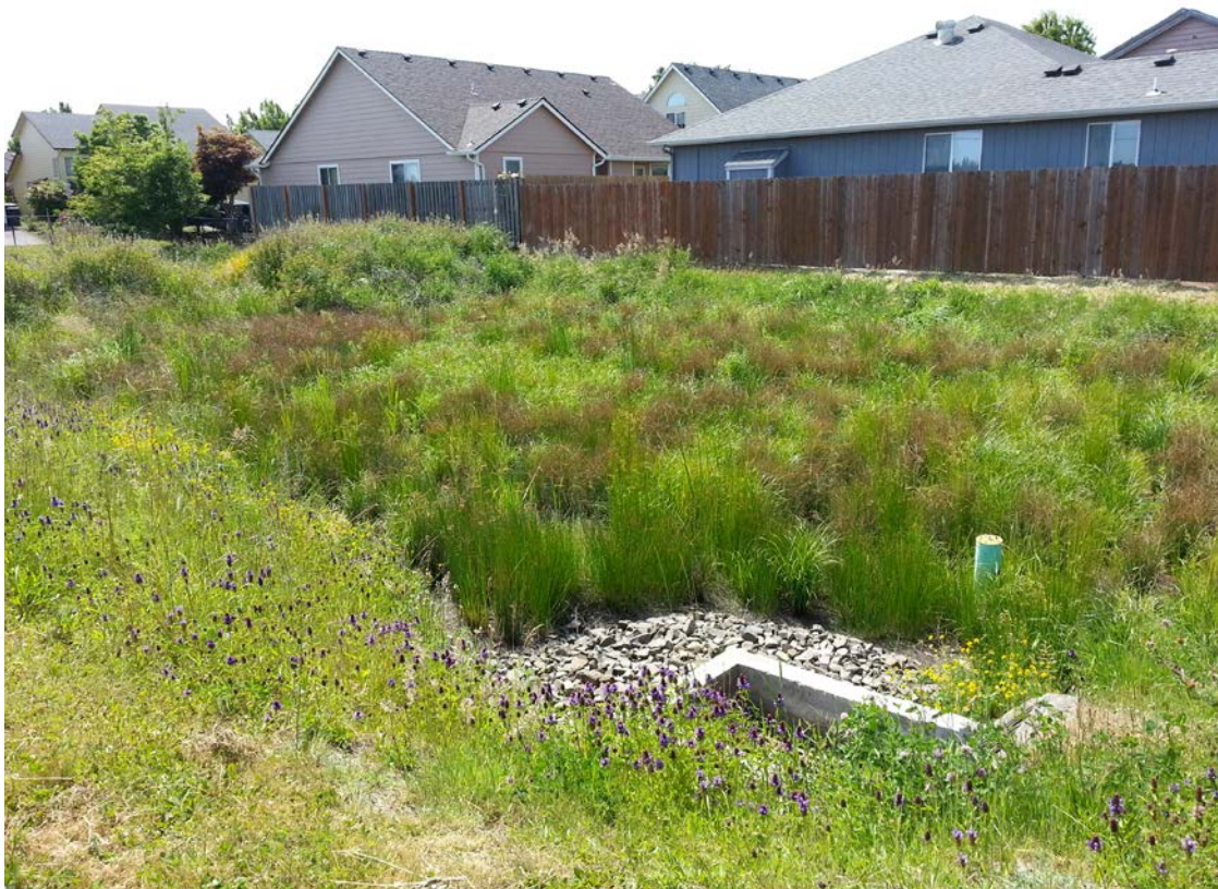
Figure 6-7. Post-construction photo of a subsurface flow wetland installed in Salem, OR.
