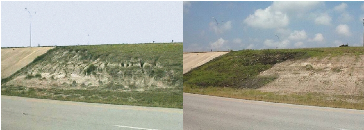
Figure 6-2. Slope erosion before and 2 weeks after erosion control compost on State Highway 47 in College Station, TX.
