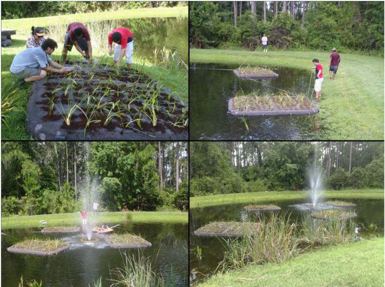
Figure 6-8. Deployment of floating wetland vegetation as a retrofit to an existing wet pond.
