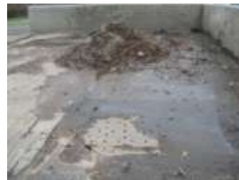
Street Sweepings Management Areas
