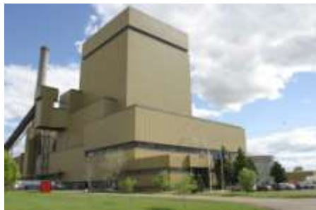
Steam Electric Power Plant
