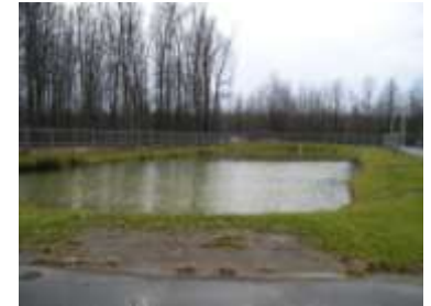
Storm Water Management Structures
