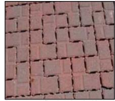
Figure 2.11.7 Pervious Interlocking Concrete Pavement
