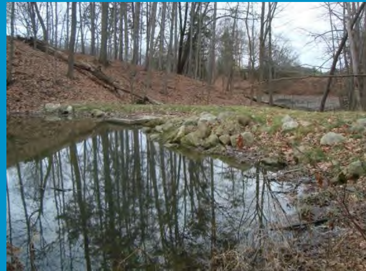
Blocked orifice, micropool, forebay
