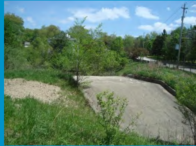
Dam, bank, or spillway erosion, blockage, woody veg
