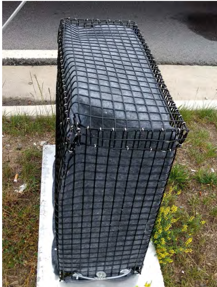
Basket was modified to fit within the catchbasin
