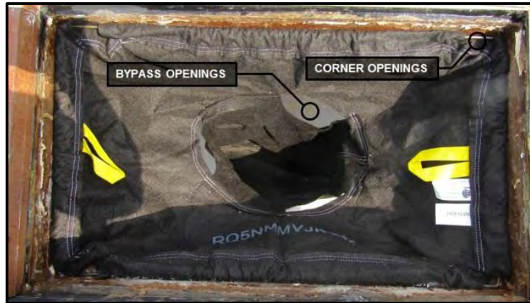
Figure C-15: Openings in Storm Sentinel® allow untreated bypass.
