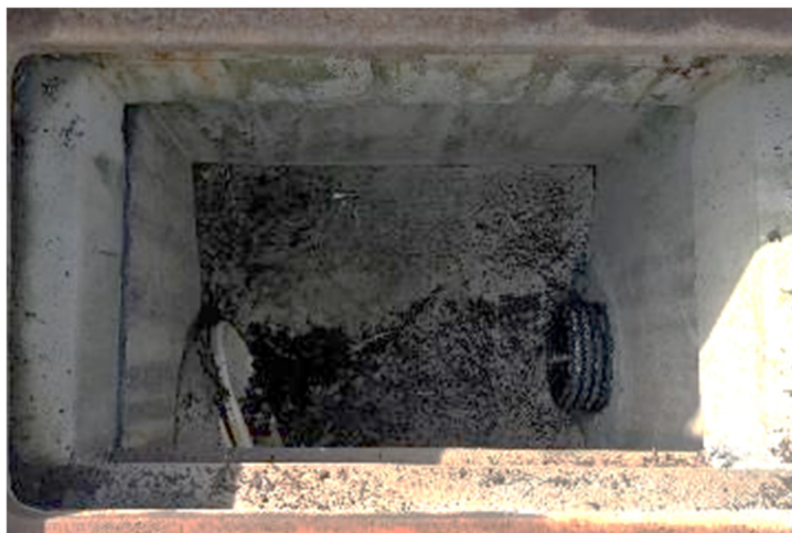
Figure 4-10 Catch Basin Connecting Conduit
