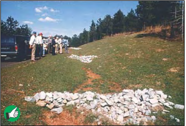
Good installation of temporary rock check dams. Remember to tie sides of check dam to upper banks. Middle section should be lower. Clean out sediment as it accumulates. Remove check dams after site and channel are stabilized with vegetation.
