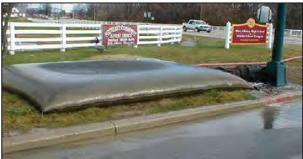
Dewatering using a sediment filter bag
