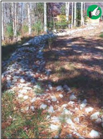
Well-built vegetated berm diverting runoff from wooded stream. Diversion berms and ditches should be seeded after construction. Use blankets if slopes are steep.
