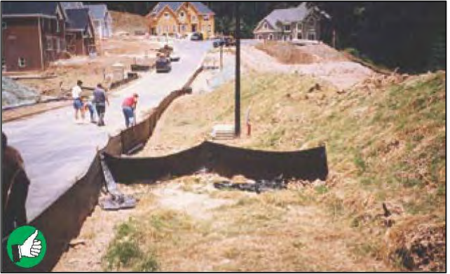
Excellent example of J-hook installation to intercept muddy runoff flowing along silt fence. Good temporary seeding and mulching (right side). Sediment must be removed before it reaches halfway to top of fence.
