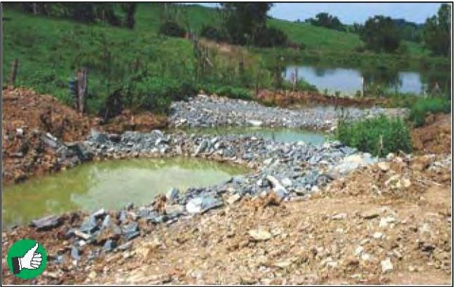
Fair installation of two traps above small pond. Dikes are a little too small; placement is too close to pond. Area needs seed and mulch.
