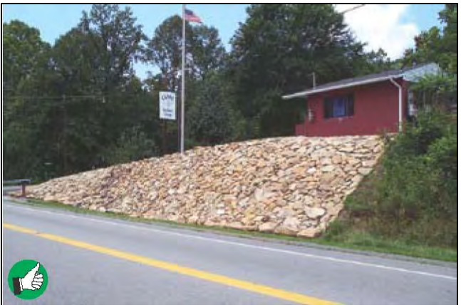
Good slope protection with permanent rock cover. This slope could have been protected with erosion control blankets or mats and seeded for a "softer" look and to promote infiltration.
