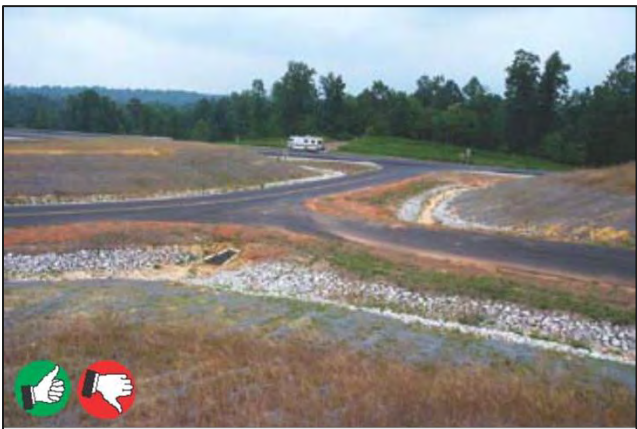
Good construction of rip-rap lined ditches on road project. Good use of erosion blankets on slopes but seed coverage on slopes is fair to poor.
