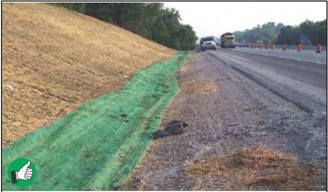
Very good installation of erosion control blanket in seeded ditch below well-mulched slope on highway project.
