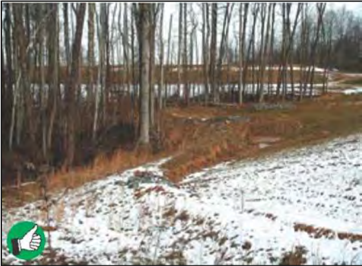
Well-built vegetated berm diverting runoff from wooded stream. Diversion berms and ditches should be seeded after construction. Use blankets if slopes are steep.
