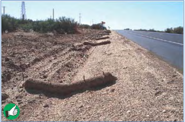
Good placement and spacing of fiber-roll check dams. Coconut fiber rolls and other commercial products can be used where ditch slopes do not exceed three percent.
