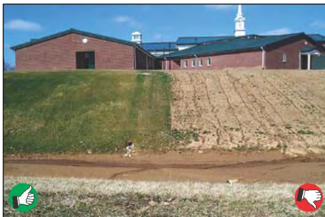
Erosion and sediment loss is virtually eliminated on seeded areas (left side). Rills and small gullies form quickly on unseeded slopes (right).
