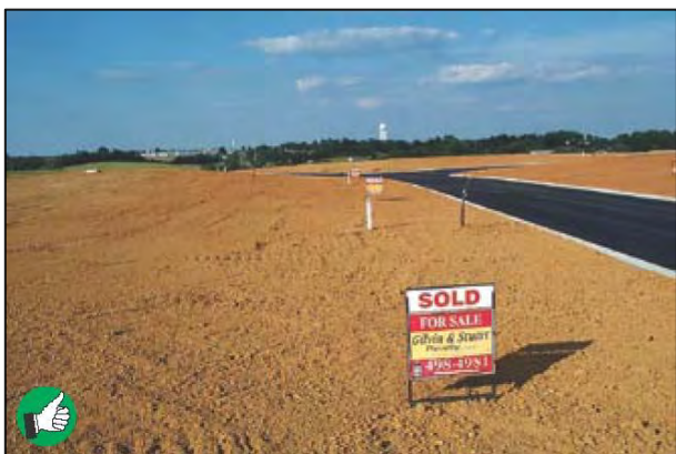
Excellent soil preparation prior to seeding. Seeded development sites erode less, are cleaner, and are easier to market than muddy sites.
