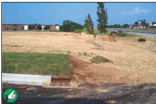
Good mix of sod, seed, and mulch at site of new community center. Note that inlet should be protected by installing a rock or sandbag berm to pond water before it flows into the inlet.
