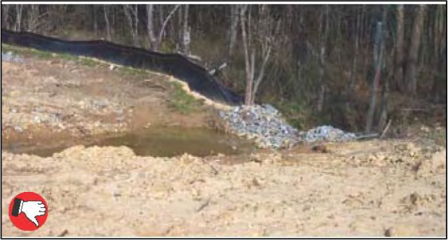
Fair to poor trap installation. Dike overflow notch is too deep; basin is too small. No seed or mulch covering bare soil areas.
