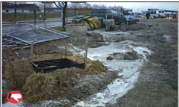
Concrete washout is not contained and debris litters the site.
