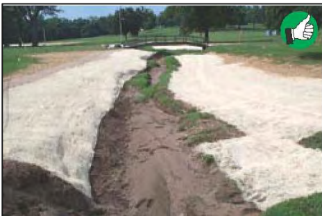
Blankets installed along stream banks or other short slopes can be laid horizontally. Install blankets vertically on longer wells. Ensure 6 inch minimum overlap.
