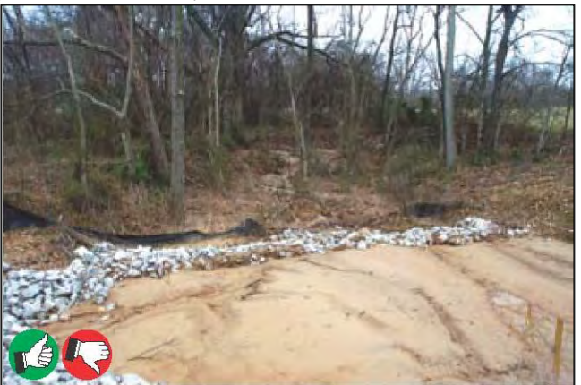
Fair sediment trap construction. Rock dike is undersized and lacks a defined overflow notch. Poor maintenance attention. Silt fence beyond rock dike is not needed—silt fence should not be used across flow channels.
