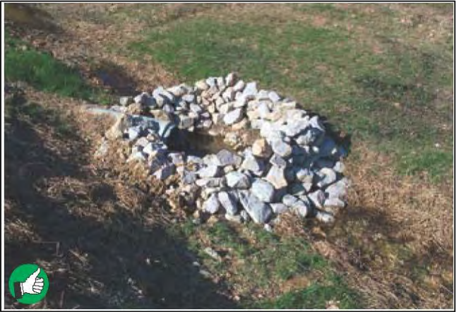
Very good application of mixed rock for culvert inlet ponding dam. Mixing rock promotes better ponding, drainage, and settling of sediment
