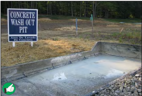
Concrete washout is properly contained
