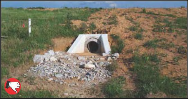
Poor rock apron placement and construction at culvert outlet; poor seeding and slope protection (right side).
