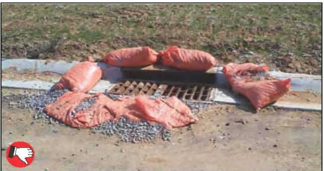
Poor placement of stone bag inlet dam; poor education of construction site drivers. Bags work well if used properly and maintained. Bags must form a dam around the inlet with no large gaps.
