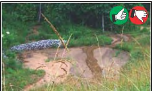
Good sediment trap installation, but poor maintenance has caused trap to fill and bypass to occur. Remove sediment before trap is half full. Make sure containment dike has an overflow notch to control the discharge location.
