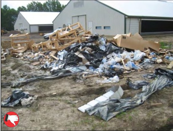
Improper storage of waste materials. Debris and contaminants can run off or blow off the site.
