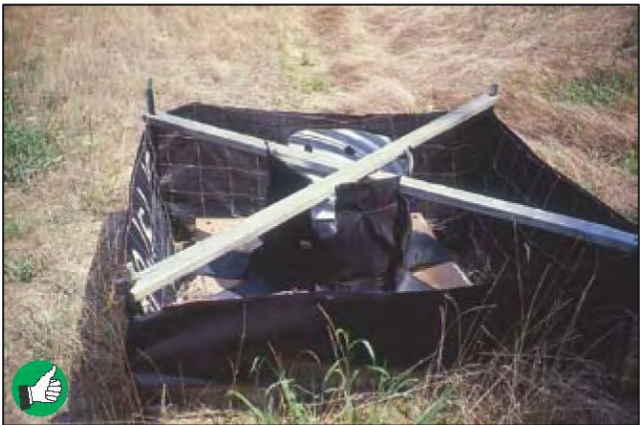
Good application of silt fence to protect drop inlet (see Section 7). Make sure fencing is trenched in and soil around fabric is compacted.
