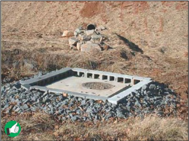
Good design and installation of inlet protection ponding dam using concrete blocks and rock. Outlet pipe in background has a rock apron to dissipate flows.
