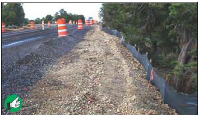
Good installation of silt fence at toe of slope. Do not pile soil or other material on silt fences. If space is available, move fence back from toe of slopes to allow room for sediment accumulation and maintenance. Leaving a strip of vegetation between bare soil and fence also improves performance.
