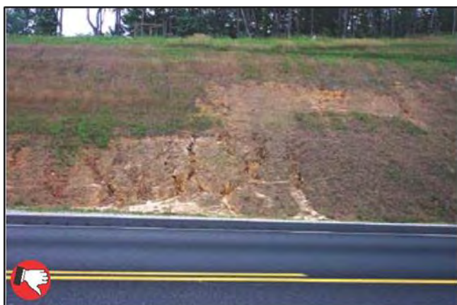
Poor seed establishment on slope. Use erosion control blankets or turf reinforcement mats when slopes are steep (greater than 4:1) and soil quality is poor. Terracing or benching steep slopes also helps.
