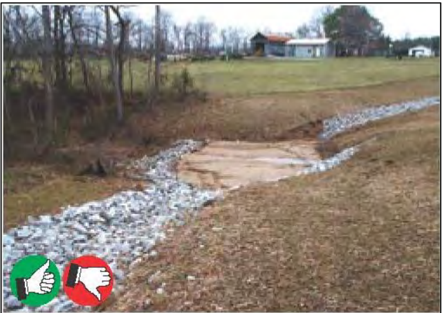
Good trap location; needs cleaning out. Trap might be too small for area drained. Very good channel protection, seeding, and mulching.
