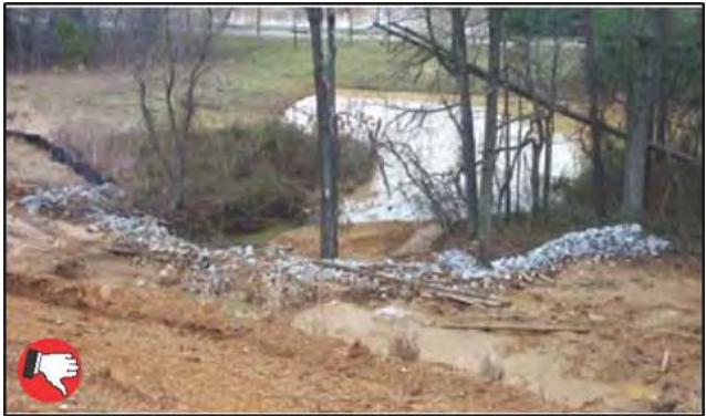
Good trap location; needs cleaning out. Trap might be too small for area drained. Very good channel protection, seeding, and mulching.
