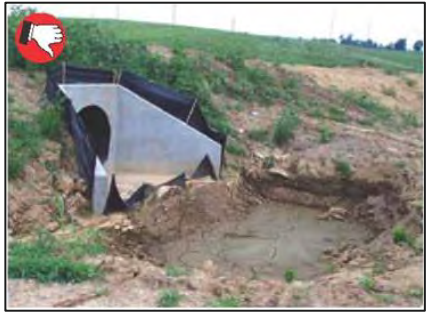
Poor rock apron placement and construction at culvert outlet; poor seeding and slope protection (right side).
