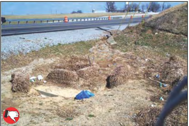
Poor protection for drop inlet on concrete pad. Straw bales make good mulch but are not suited for inlet protection or silt check dams.
