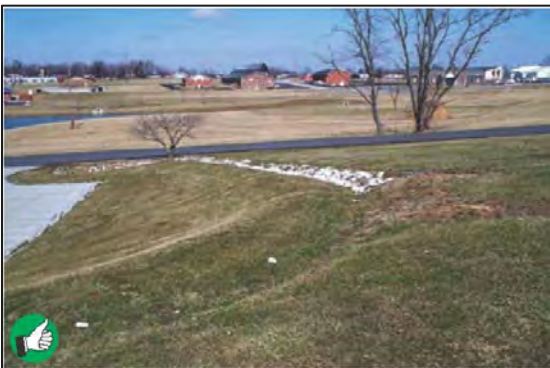
Good example of construction, seeding and stabilization of diversion berm. Note that diversion ditch is lined with grass on flatter part of slope, and with rock on steeper part.
