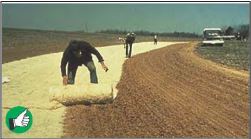
Blankets installed along stream banks or other short slopes can be laid horizontally. Install blankets vertically on longer wells. Ensure 6 inch minimum overlap.
