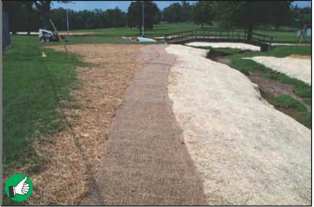
Excellent soil coverage at stream bank stabilization project using hand scattered straw, jute matting, and erosion blanket.
